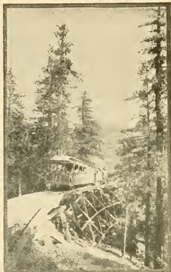
HIGH-CURVE TRESTLE, MT. TAMALPAIS RAILWAY.
